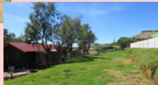
建設中の簡易宿泊施設(左)とフェンス(右) Construction of the simple accommodation facility is underway (left) and the park fence (right)
