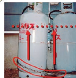
An example of a chain that is dangerous because it is loose
